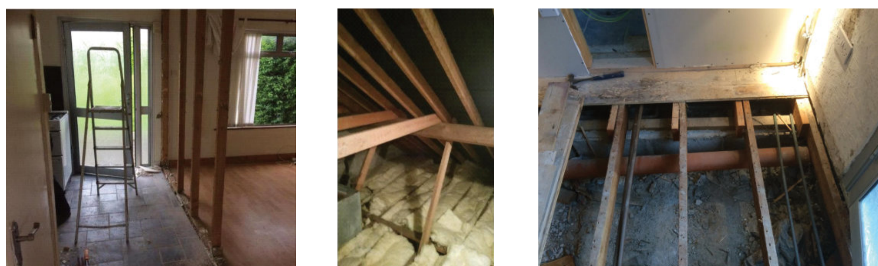
Figure 5: Case Study; Typical Suburban Semi-Detached House - Survey / Demolition Photos
