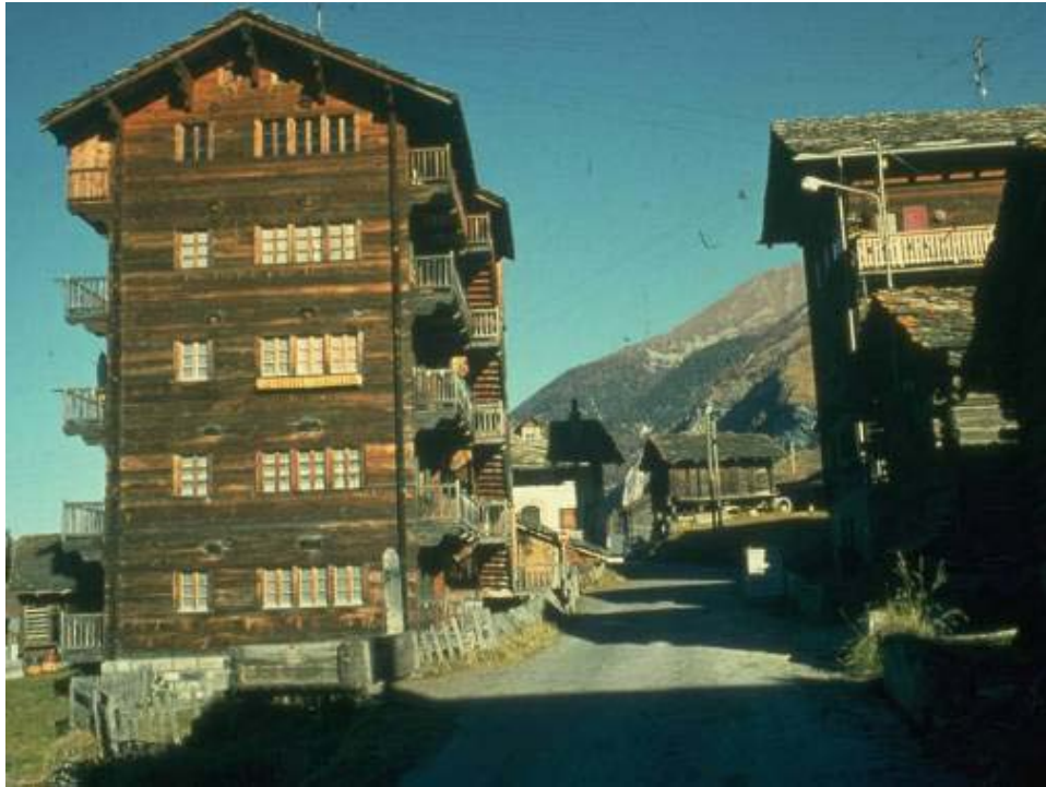
Multi-storey log construction, CH-Valley
