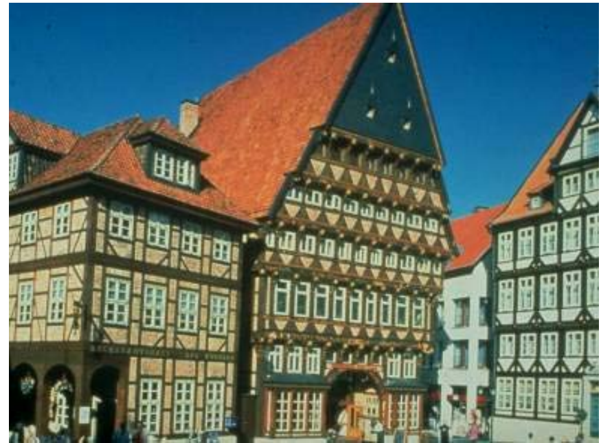
Multi-storey timber frame construction, De-Hildesheim
