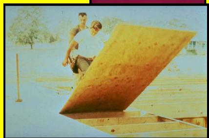
Perhaps you listed particleboard. This is a product made by gluing small flakes, shavings, or splinters of wood together using heat and pressure to form larger panels.
