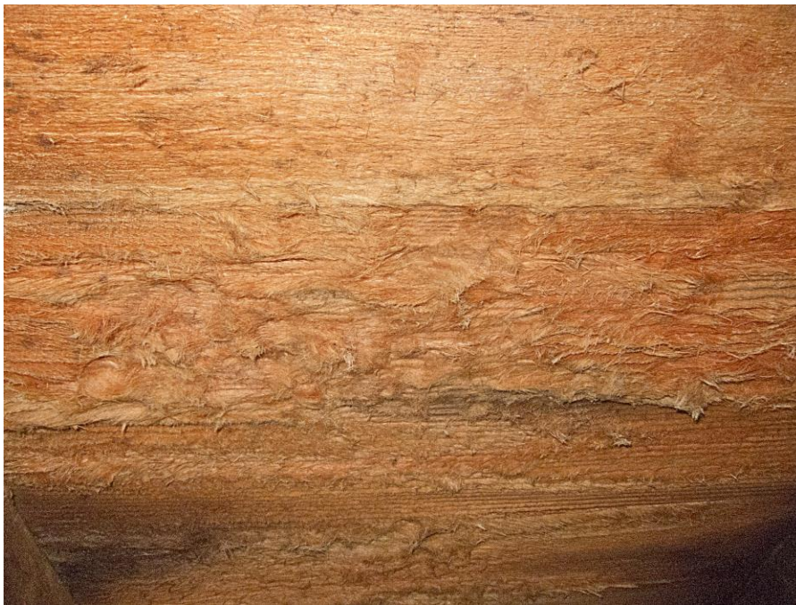
Figure 27. Salt-damaged wood on Mayflower II. This photograph was taken from the underside of a porch (cubbridge head) where the people exit from between decks, at the middle level of the ship.
