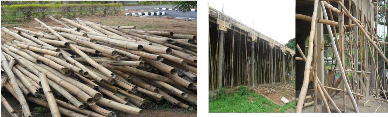
Plate 3.1: Mode in which Recovered Bamboo Culms from Scaffold is Stored
