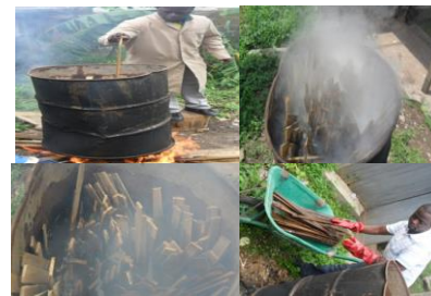
Plate 1.1: Treating Bamboo Strips
