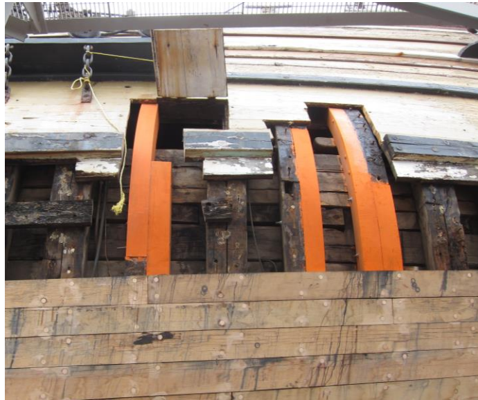
Figure 25. The orange paint is a protective marine coating used on the new futtocks installed on the port side of the Mayflower II at Fairhaven Shipyard. Note the new white oak planking.
