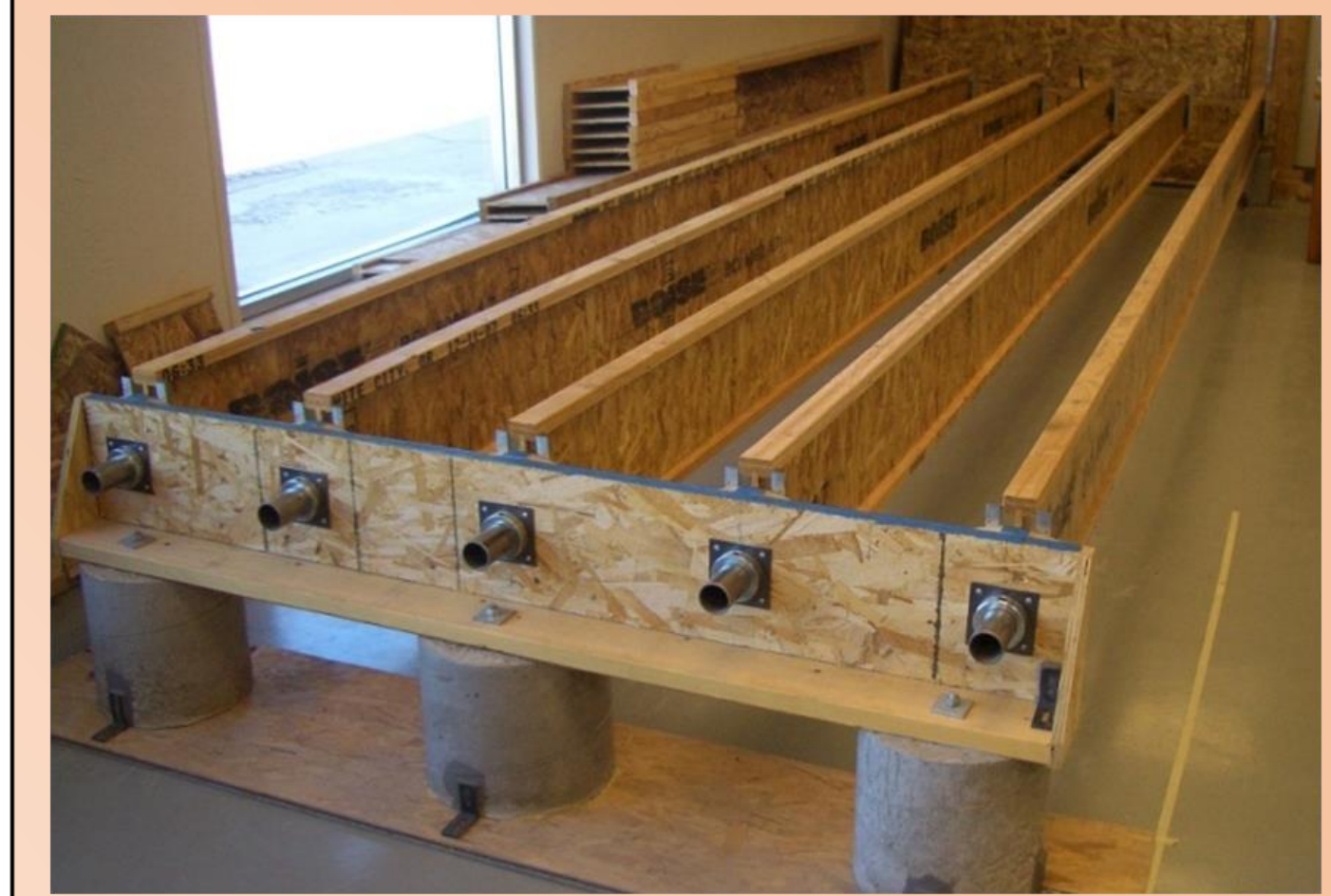
Figure 3. Wolfe's floor without sheathing
