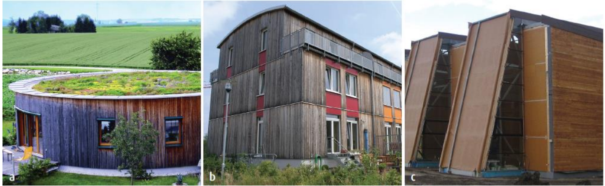
Fig. 5 Different types of passive houses: (a) Single family passive house, (b) Multy storey timber frame passive house, (c) Industrial building.
