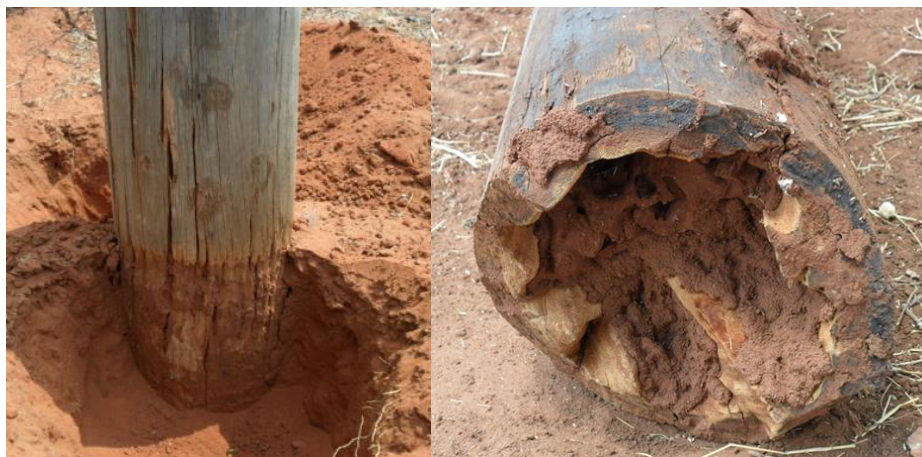
Figure 4: Typical degradation observed on electricity transmission wood poles
