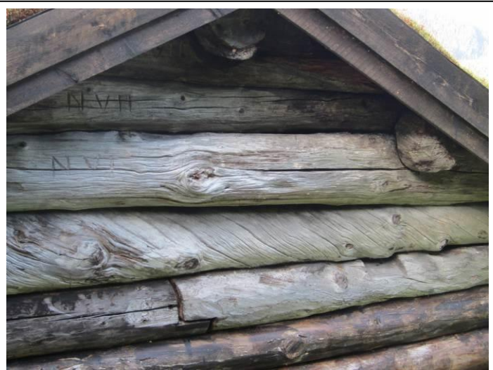
Fig. 1 A log with heavily twisted grain included in a loghouse construction along with more straight-grained logs.
