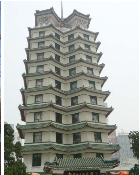
pseudo-classic building constructed of reinforced concrete 钢筋混凝土仿古建筑
