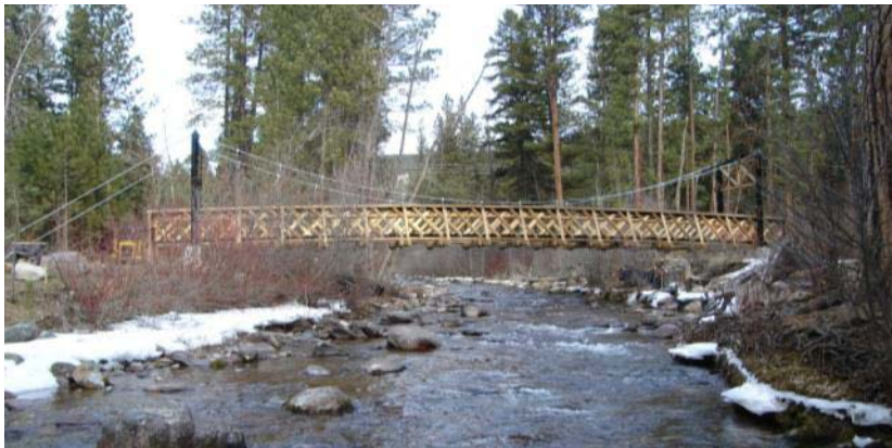
Rattlesnake Creek bridge, Missoula, Montana
