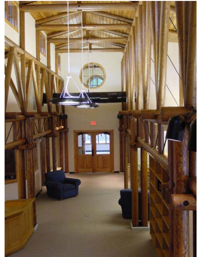
Six-inch-diameter lodgepole pine used in 5,000 ft 2 library in Darby, Montana.
