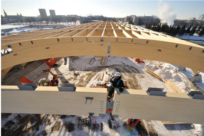
Assembly and installation of main arches
