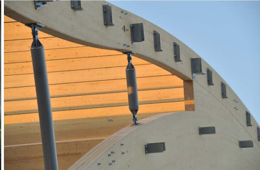
Hybrid structure under construction
