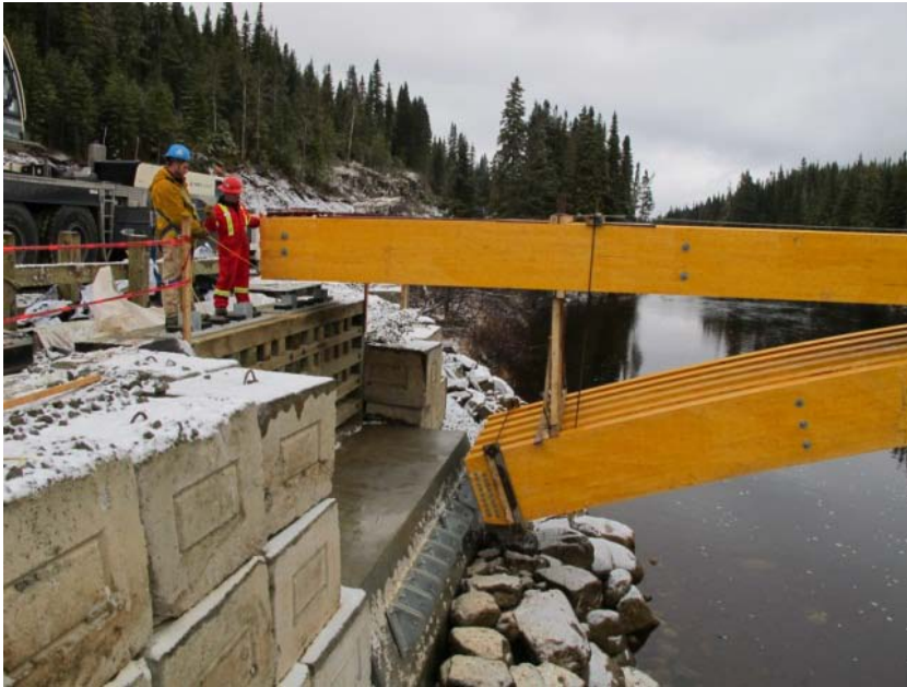
Installation of bridge section and connectors to concrete base
