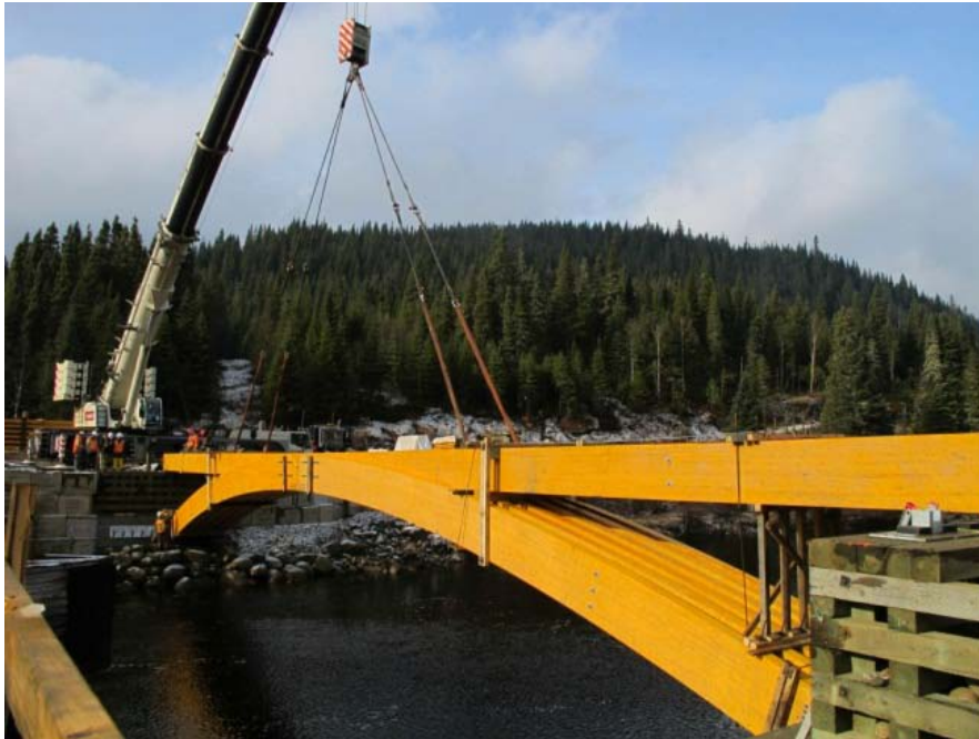
Installation of bridge section
