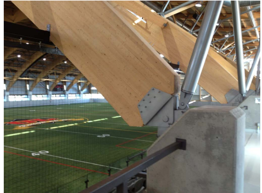
Glulam connectors to concrete base
