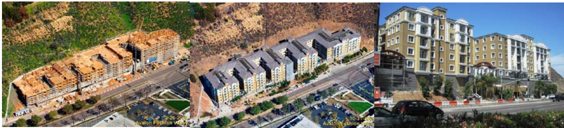
Figure 2 Fashion Walk: 5 stories of wood frame over two levels of exposed concrete parking. A seven-story building utilized a sloping site to pick up an additional story. Photos courtesy of Tim Smith, President, Togawa Smith Martin, Inc.
