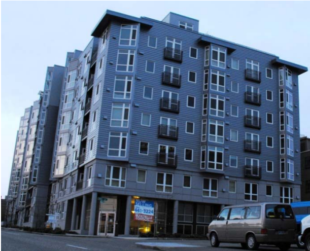
Figure 8: Marselle Condos in Seattle, Washington – a 160,000 square foot condo project of IBC Type III construction has five floors of wood construction over a two-story concrete podium construction.
