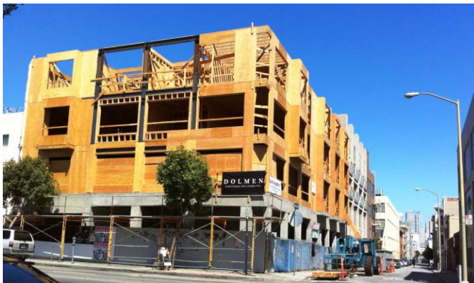
Figure 7: Podium Construction in San Francisco, California in 2010
