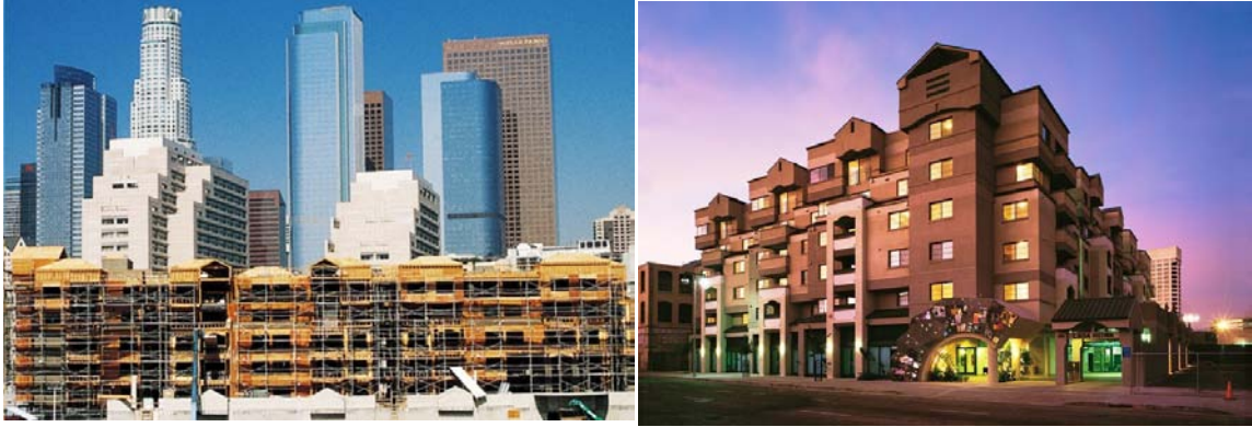
Figure 5 Casa Heiwa: A 5-story wood framed building in California, built in 1995, achieved high density of 100 units per acre. Photos courtesy of Tim Smith, President, Togawa Smith Martin, Inc.
