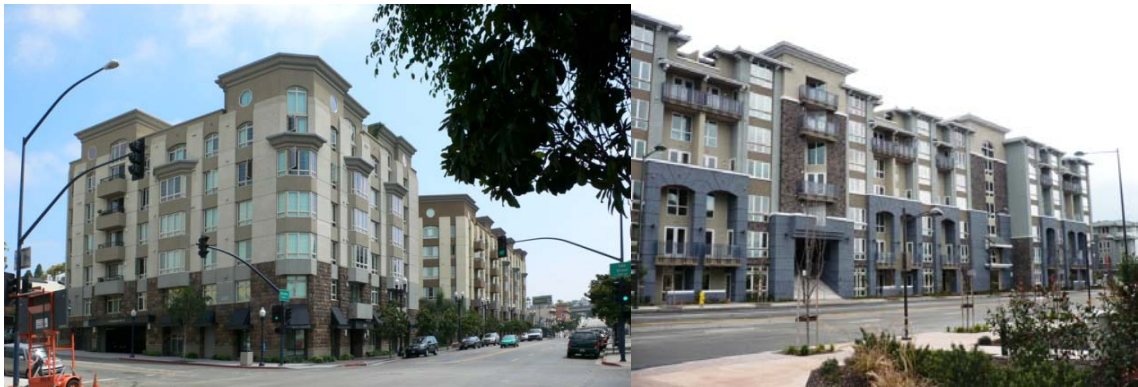
Figure 6 Union Square & Elan: 7 levels residential building - one level of concrete and 6 levels of wood framing. Density of 130-140 units per acre. Photos courtesy of Tim Smith, President, Togawa Smith Martin, Inc.
