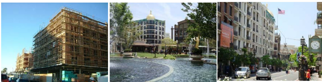
Figure 4 Americana: 5 story wood frame over one story retail podium of concrete construction. A typical European infill project creating high density housing with active retail base designed for 100 units per acre. Photos courtesy of Tim Smith.
