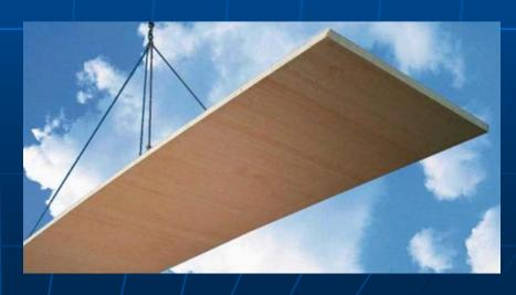
Each element is prefabricated with given length, width and openings for windows, doors, stairs etc.
