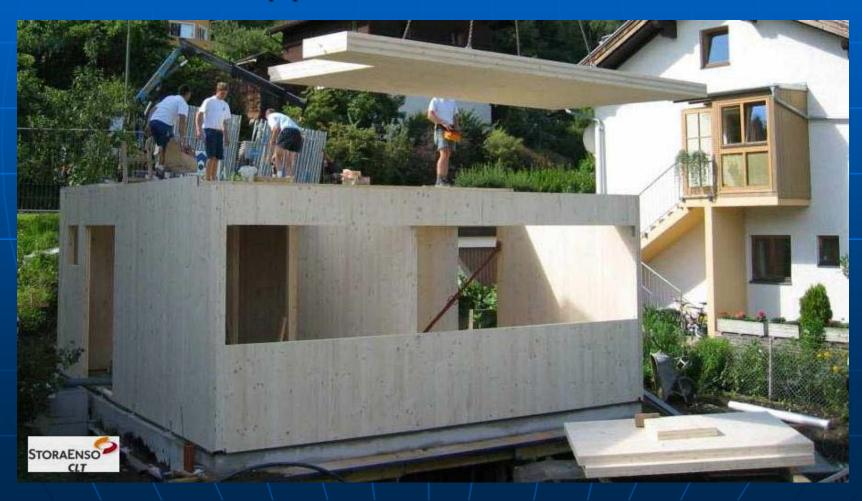
The panels are dimensionally stable and fire retardant, strong mechanically and low in thermal conductivity.
