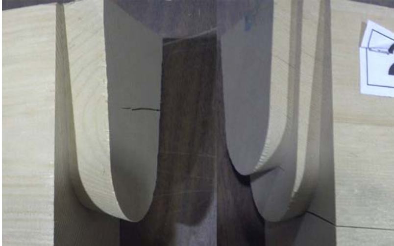
Figure 1: Single (left) and double rounded dovetail joint (right)
