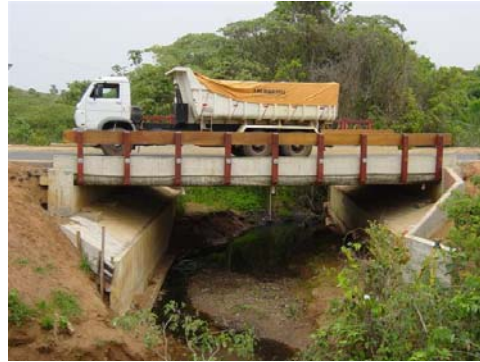
Fig. 6 - The completed P01 Bridge
