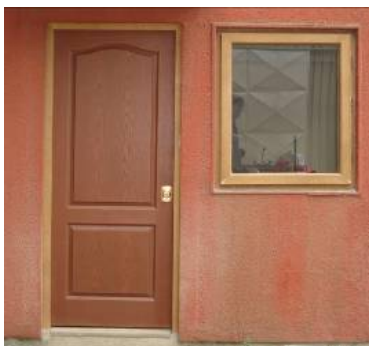
Figure 4. Wood-plastic door and window installed in a pilot house, Universidad del Bío-Bío.
