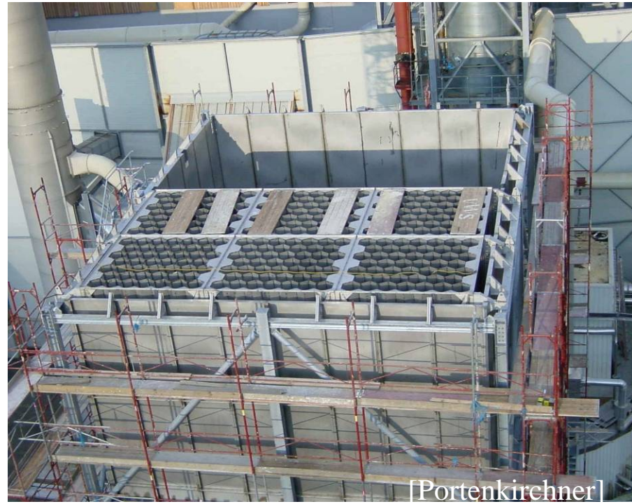
Wet electrostatic precipitator
