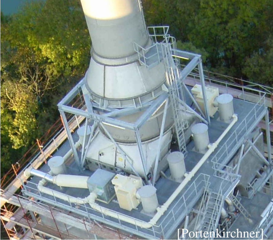
High voltage unit
