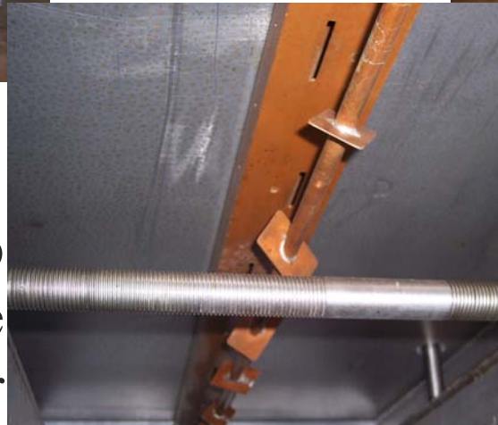
Top Microwave Radiator
